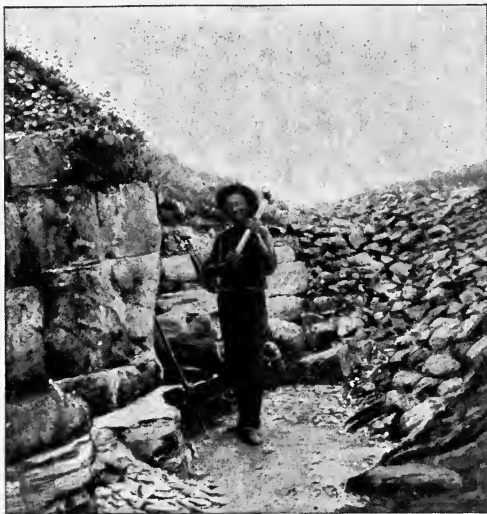
INDIAN QUARRYMAN OF TO-DAY. THE PIPESTONE LEDGE APPEARS AT THE BASE OF THE WALL. (BENNETT, COLL.)
